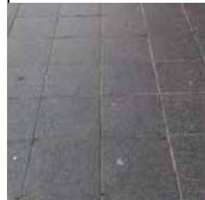
Standard gun metal stone pavers in the commercial area
