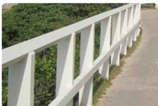
Coast Walk timber railing
