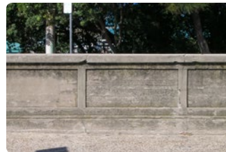
Boundary wall along Campbell Parade
