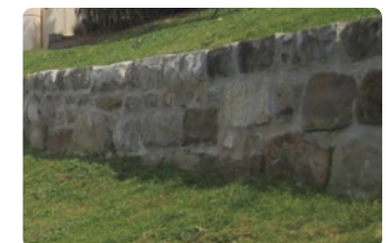
Sandstone retaining wall
