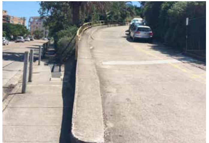
Image: There is limited wayfinding signage
