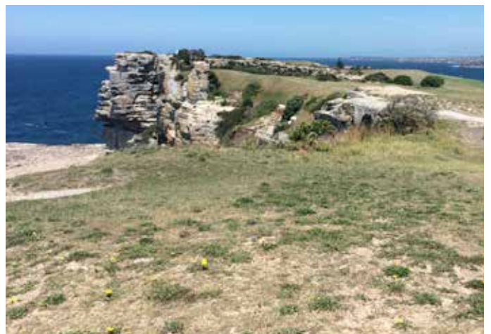
Image: Access to the cliff edge is un-restricted
