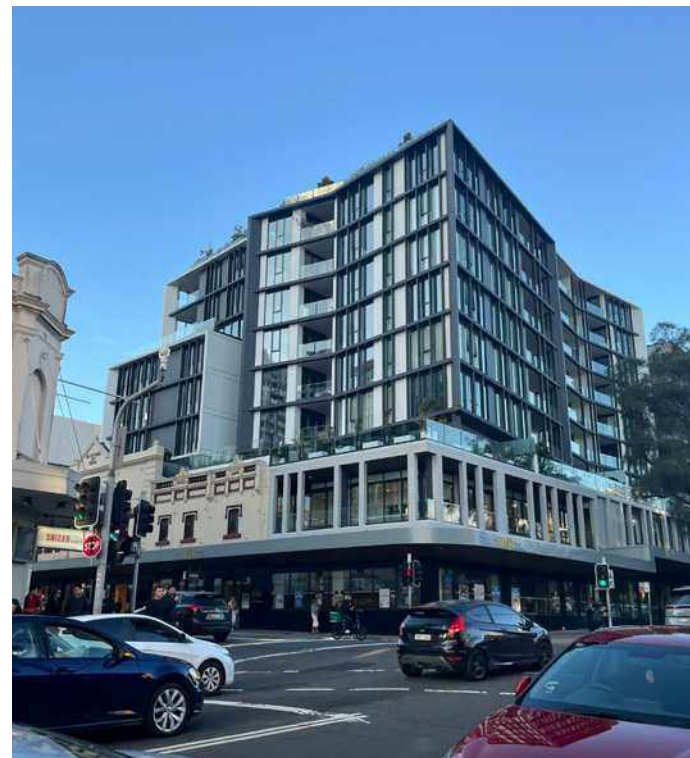
⑥ 28-38 Bronte Road, constructed in 2024. 8 storeys
